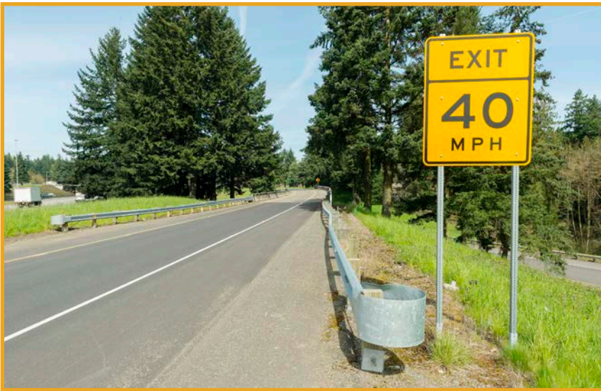
Above: The I-5 north Charbonneau exit ramp south of the Boone Bridge.
